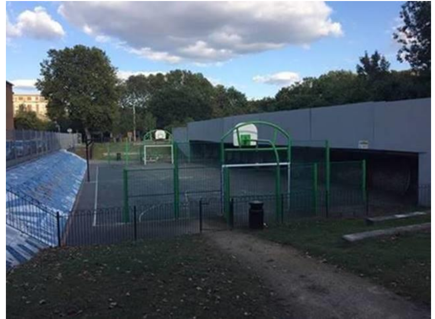
existing pedestrian bridge (right) demolished due to structural issues since August 2022
